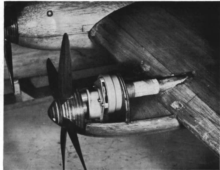
Mk. IIb turbine installed in nacelle
