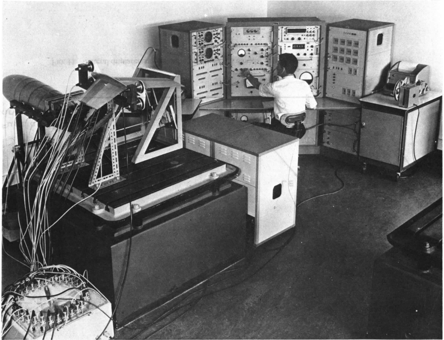
FIG. 10. Resonance testing of the flutter model.
